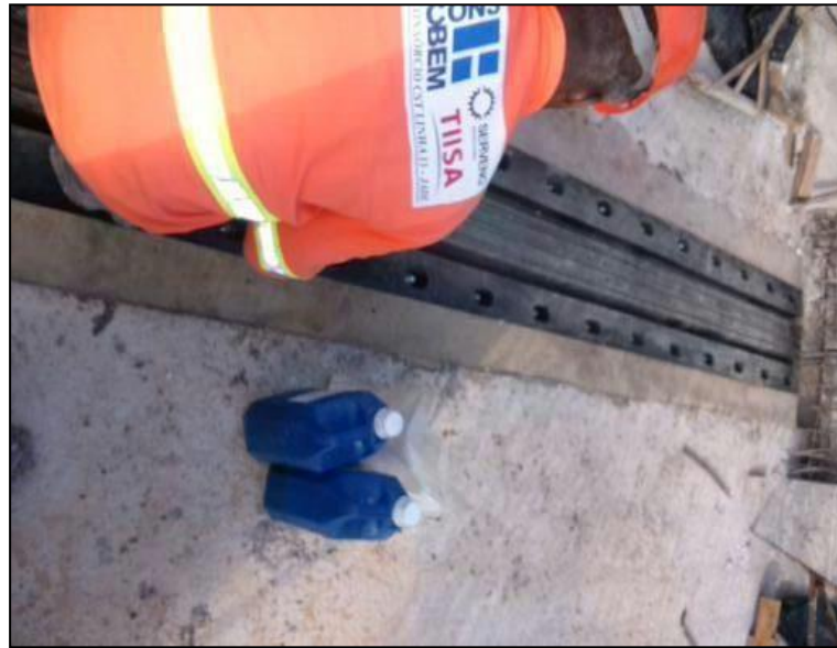
Figure 12 - Junta NP 160 Instalada
