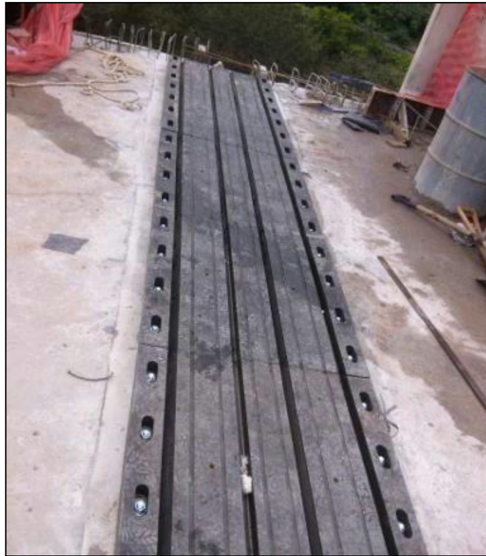
Figure 15 - Junta NP 260 Instalada
