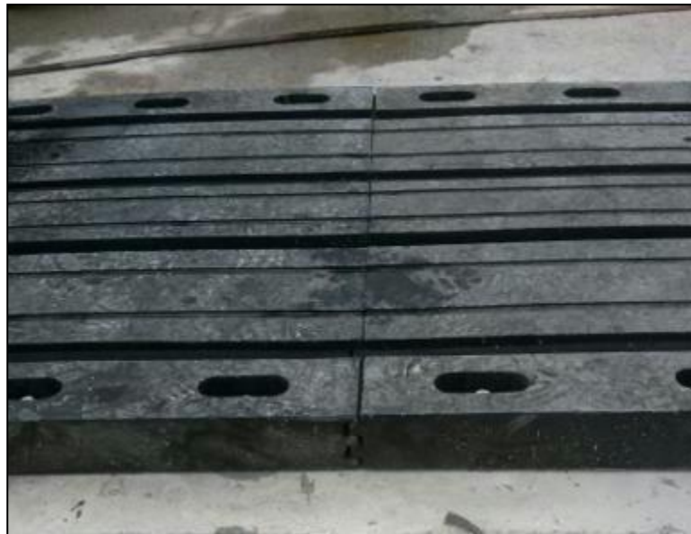
Figure 12 - Junta NP 160 Instalada
